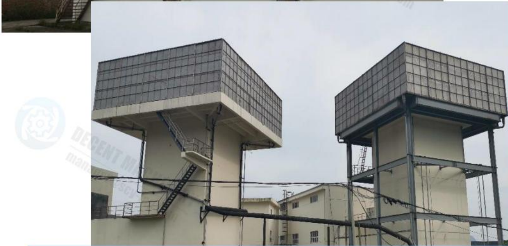
Dust Removal Transformation of Fan Outlet in Fankou Lead Zinc Mine
