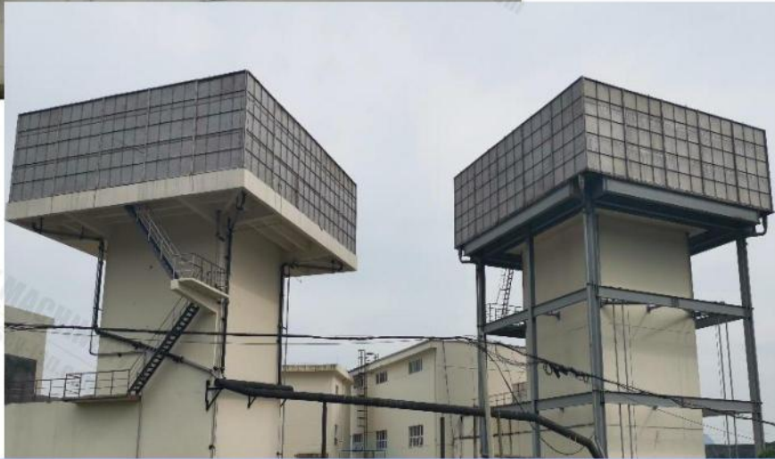
Dust Removal Transformation of Fan Outlet in Fankou Lead Zinc Mine
