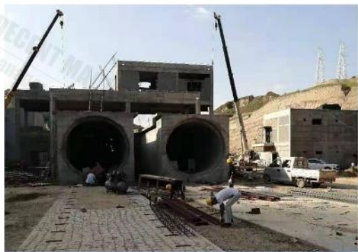
EPC Installation: FBCDZ - No 28 main fan of Yan'an Hecaogou Coal Industry Co., Ltd
