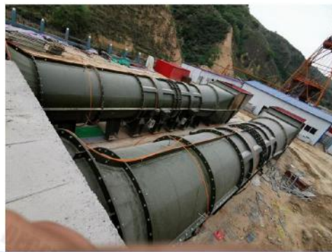
EPC Installation: FBCDZ - No 28 main fan of Yan'an Hecaogou Coal Industry Co., Ltd
