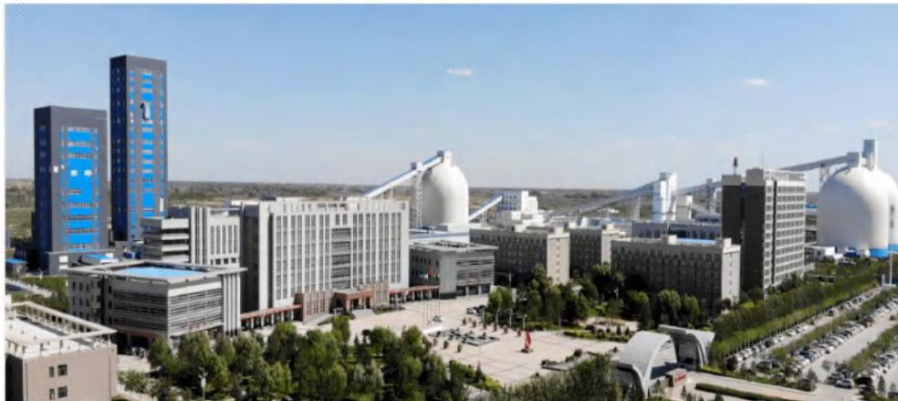
Zhongtian Hechuang Mengkeqing Coal Mine Intelligent remote Centralized Control System For Ventilation
